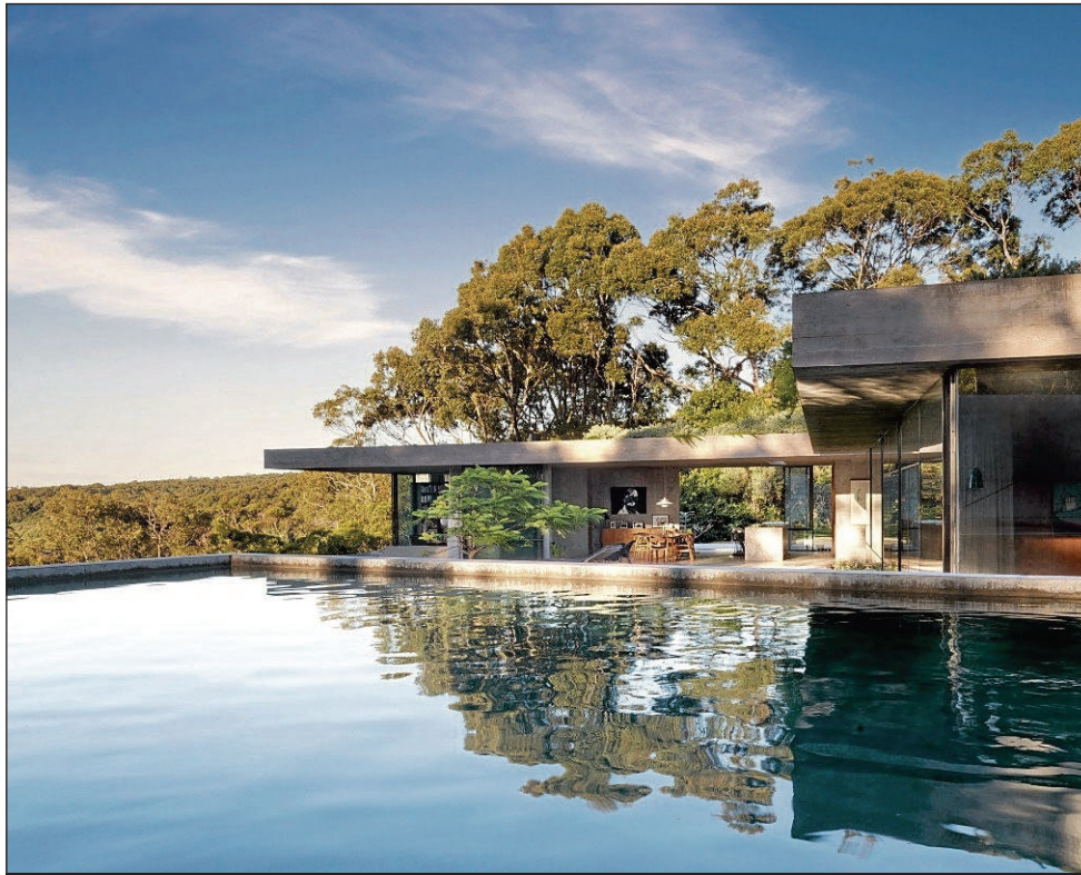
SYMBIOSIS OF ARCHITECTURE AND NATURE: Embedded in the hillside on Burwood Road, the 'Bunkeren', built by Ledbury Constructions, collects its own water and makes its own power and heat and has net zero emissions.
